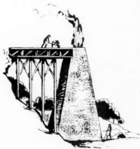
And how!! Early Iron Furnace in operation.
